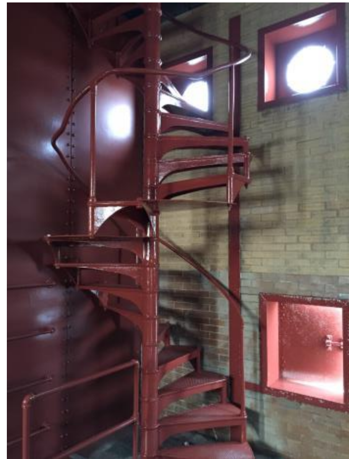
Inside Staircase Post NCP SiloxoSheild 2K
